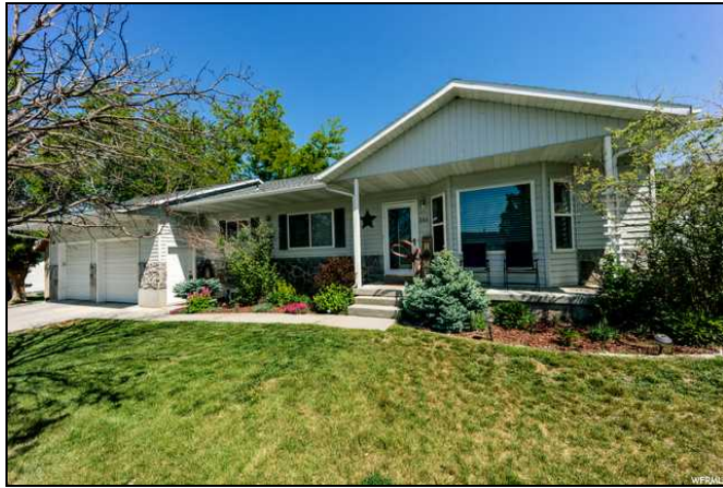
Front of Home: Home is South Facing
